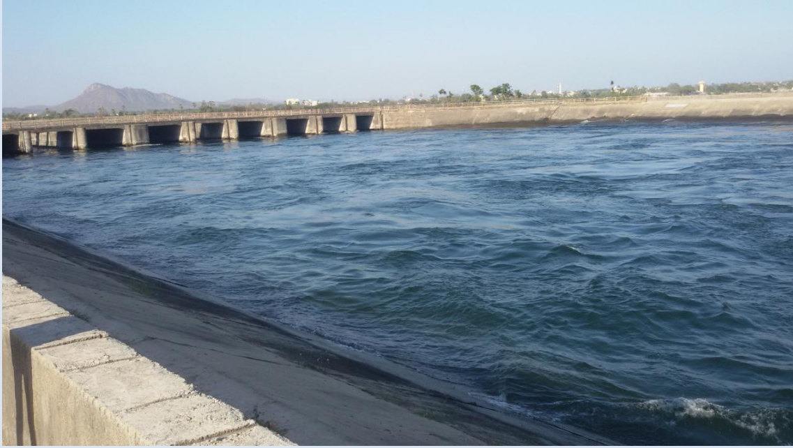
Fig. 4 Syphon Aqueduct on Orsang river at Bodeli
