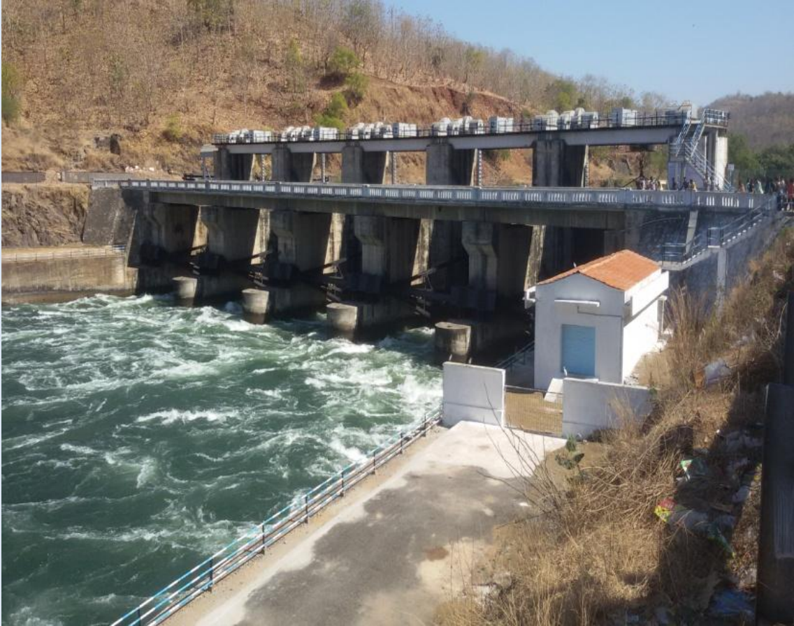
Fig. 2 Narmada Main Canal Gate
