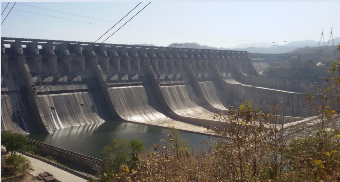
Fig. 1 Sardar Sarovar Dam
